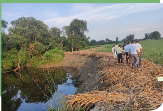
Village Budhapurva Block Palia 3200 mtrs bund repair work
