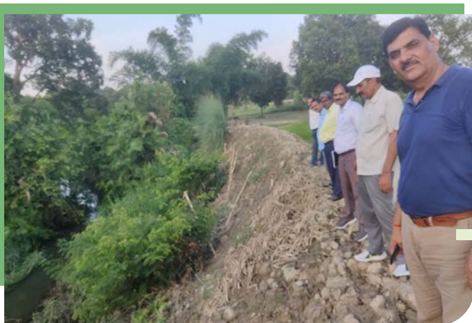
Village Gola-block Palia 90 mtrs bund repair work
