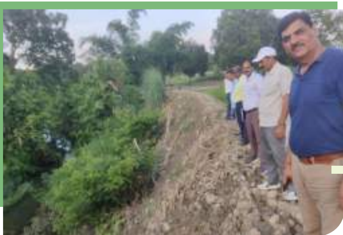
Village Gola-block Palia 90 mtrs bund repair work
